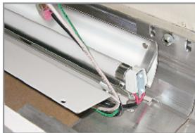
1. insert preassembled luminaire
